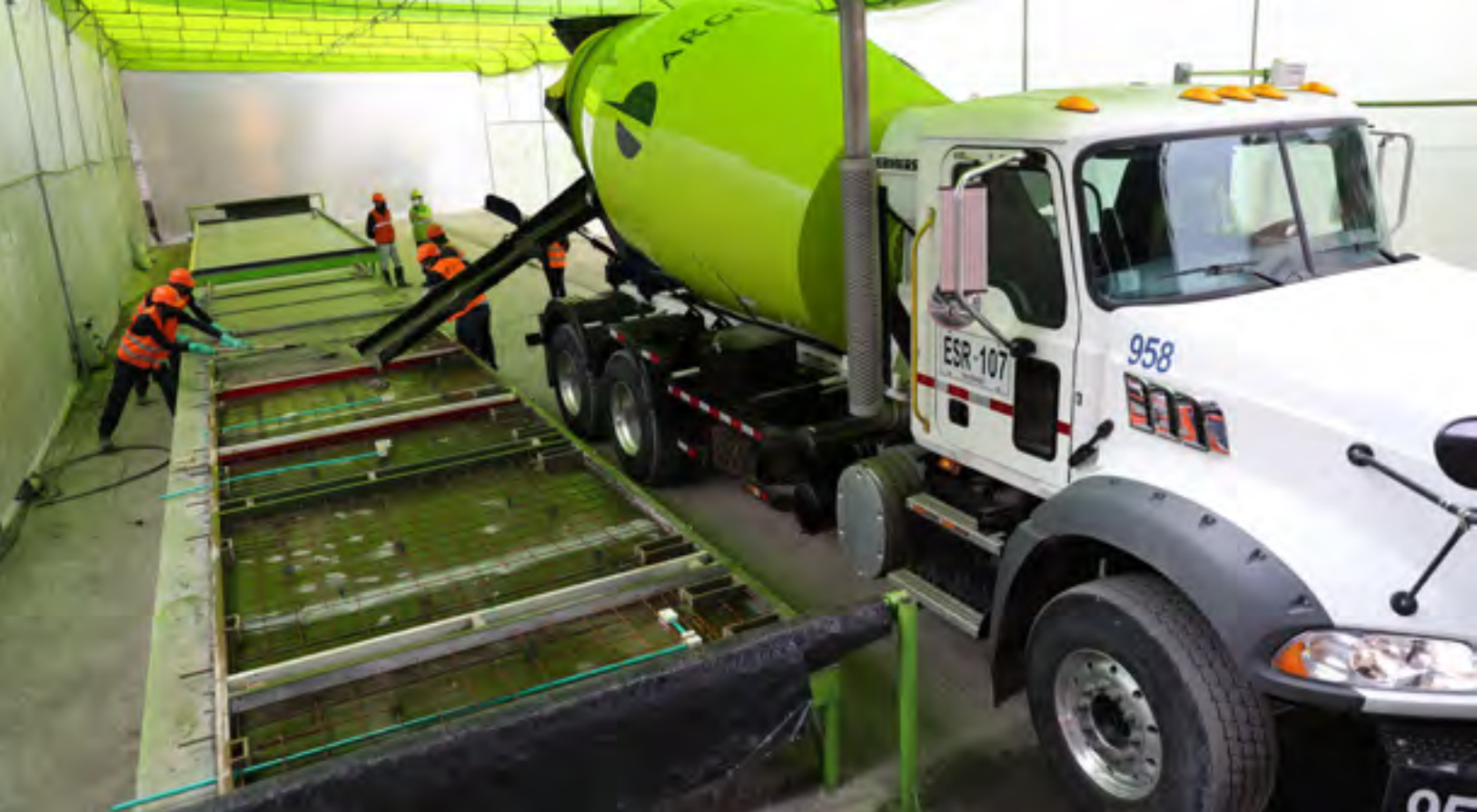
↑ Production of precast concrete modular panels
