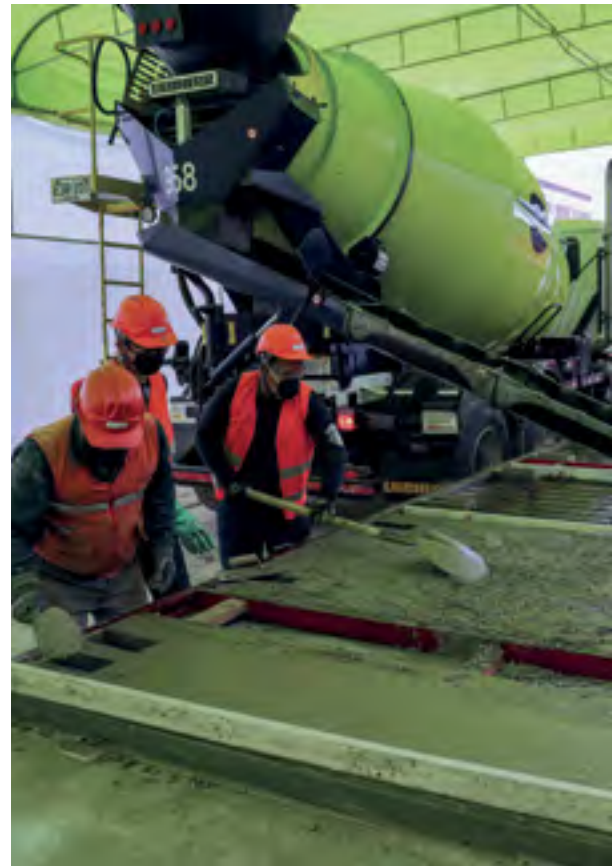
↑ Production process of concrete modules
