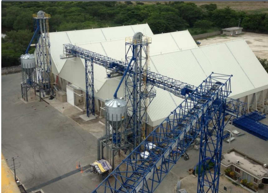
Bulk plant in Tolú
