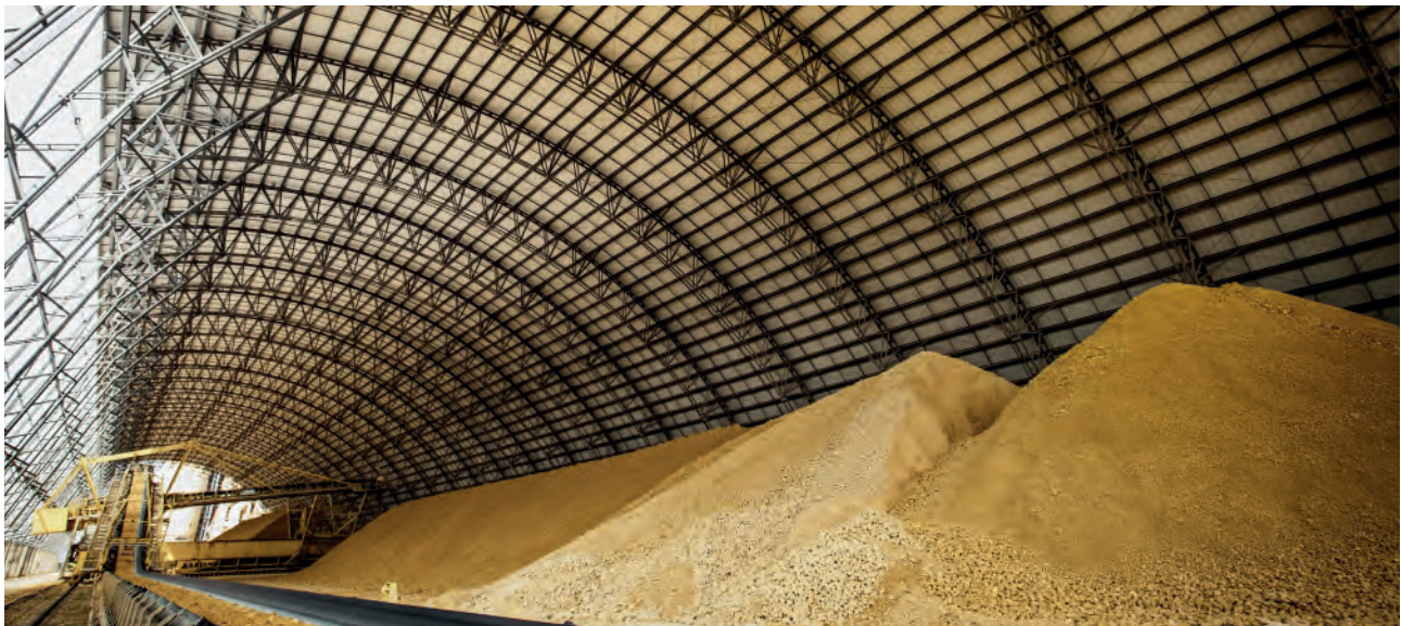
Cartagena Plant - Cementos Argos Bolívar, Colombia.
