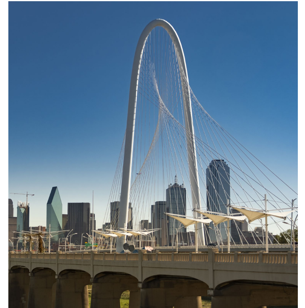
▶ Margaret Hunt Hill Bridge, work with Argos seal United States
