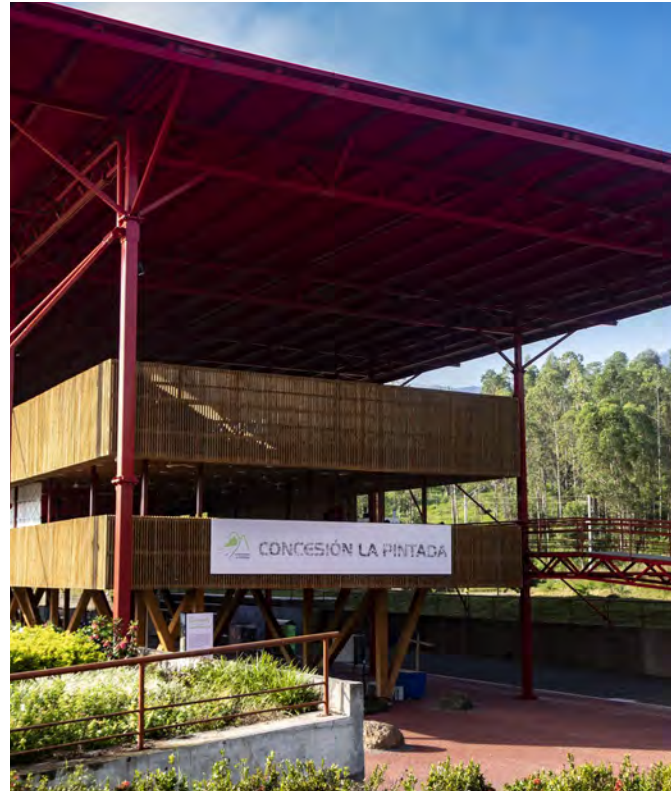
Pacifico 2 Operations Control Center Antioquia
