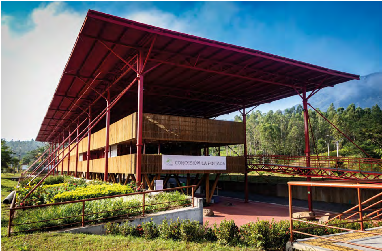
Pacifico 2 Operations Control Center Antioquia
