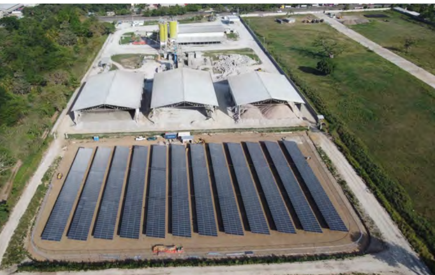
Solar farm of the Cementos Argos Choloma plant Honduras
