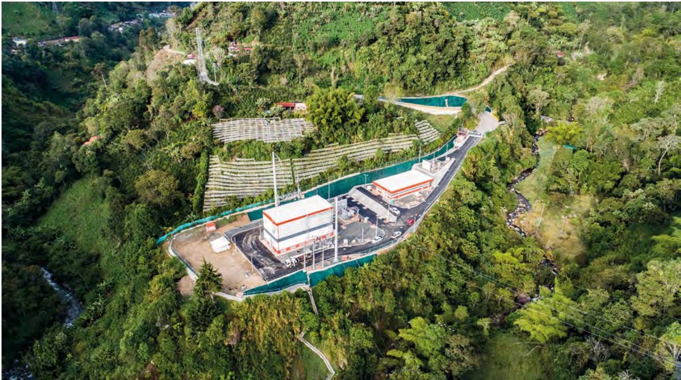
Cajamarca Substation Tolima
