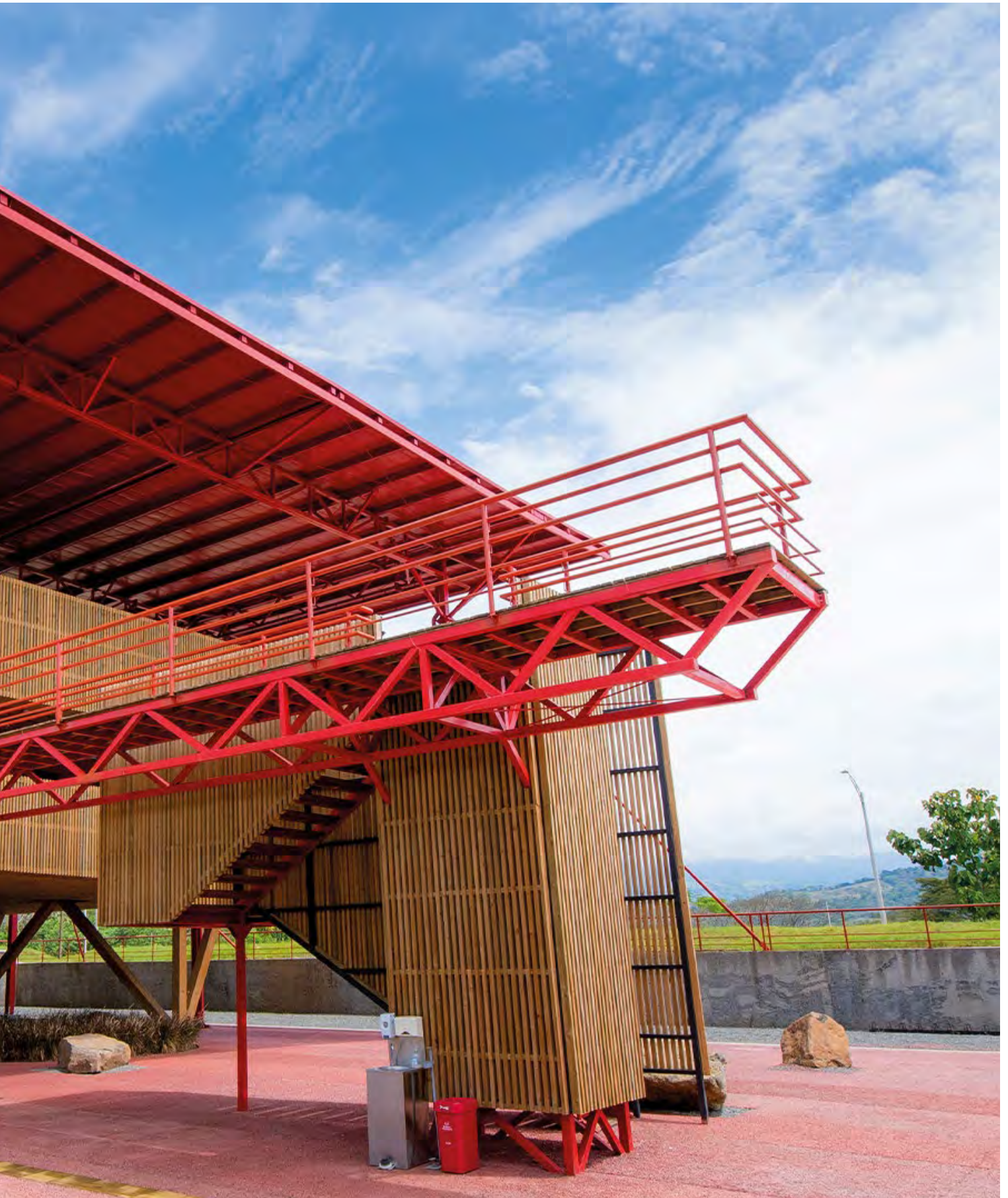
Pacifico 2 Operations Control Center Antioquia
