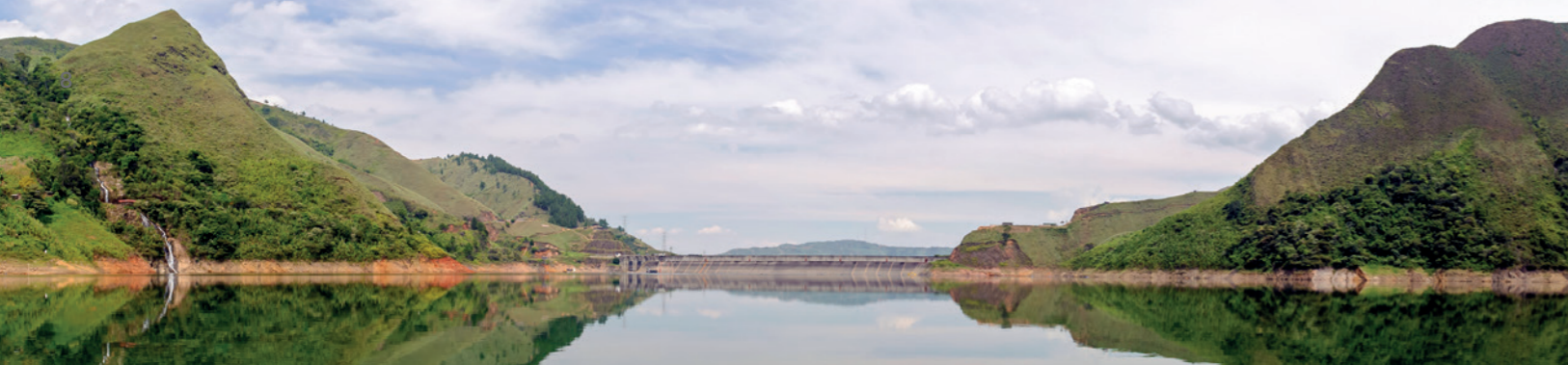
▶ Salvajina Hydroelectric Plant Cauca
