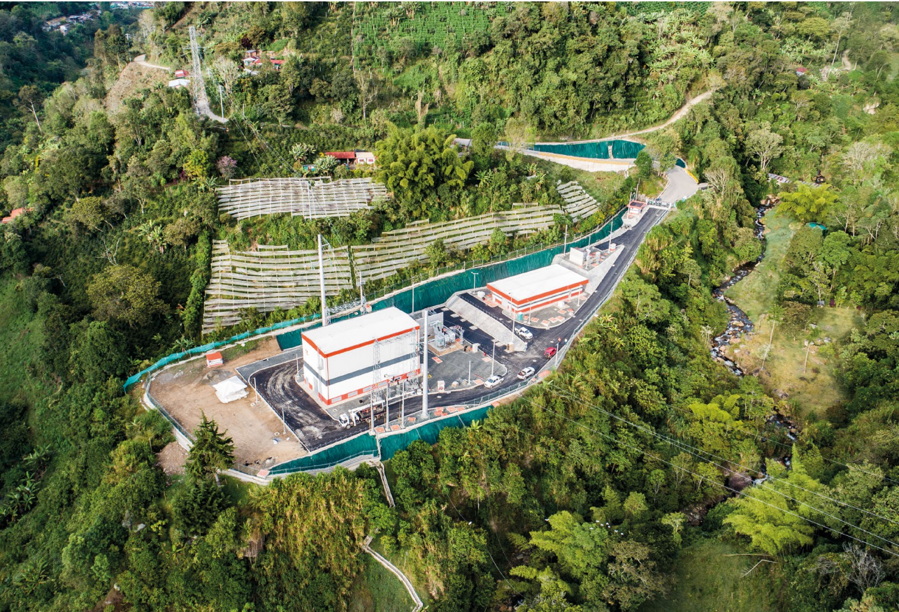
Cajamarca Substation Tolima
