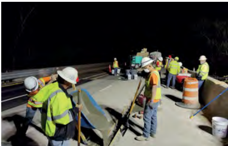
↑ Construction with UHPC Concrete; the United States
