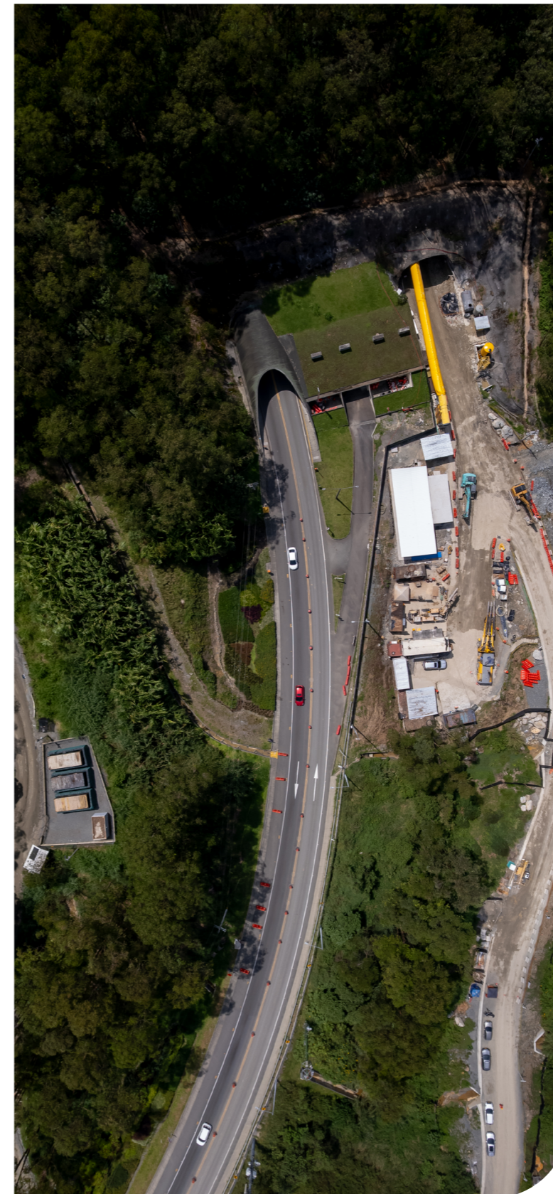
Construction for the second stage of Túnel de Oriente, Antioquia
