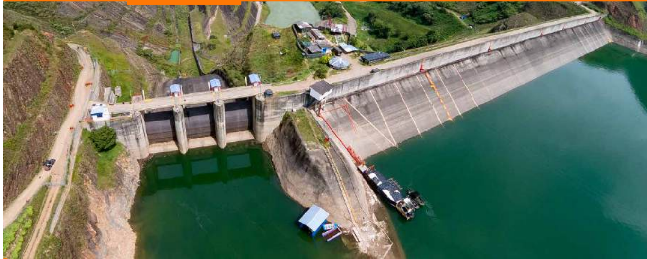
Salvajina Hydroelectric Plant, Cauca
