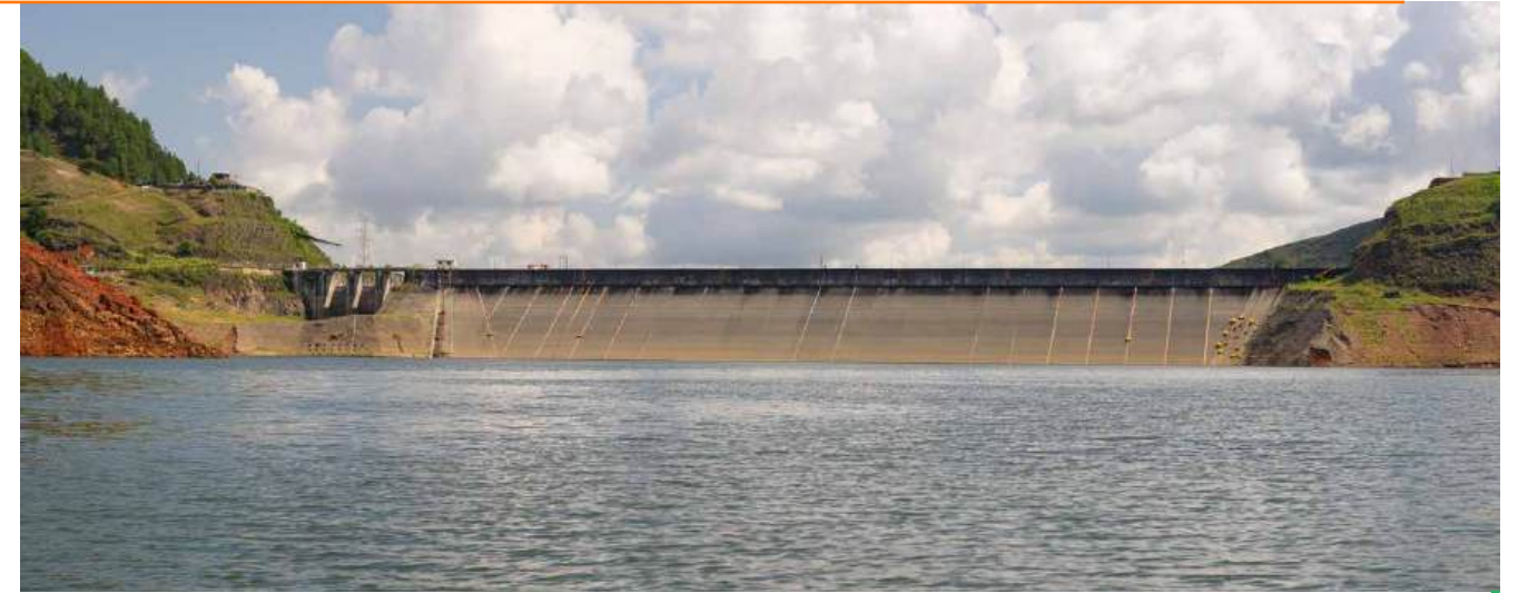
Salvajina Hydroelectric Plant, Cauca.
