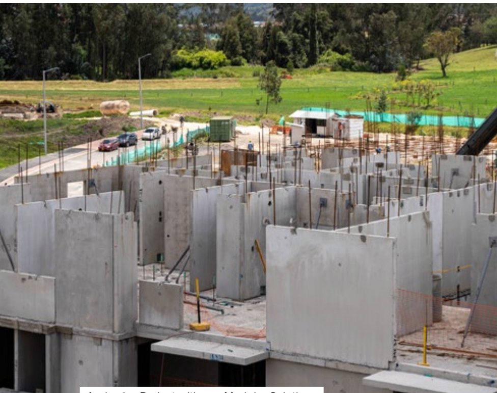
Andarríos Project with our Modular Solutions
