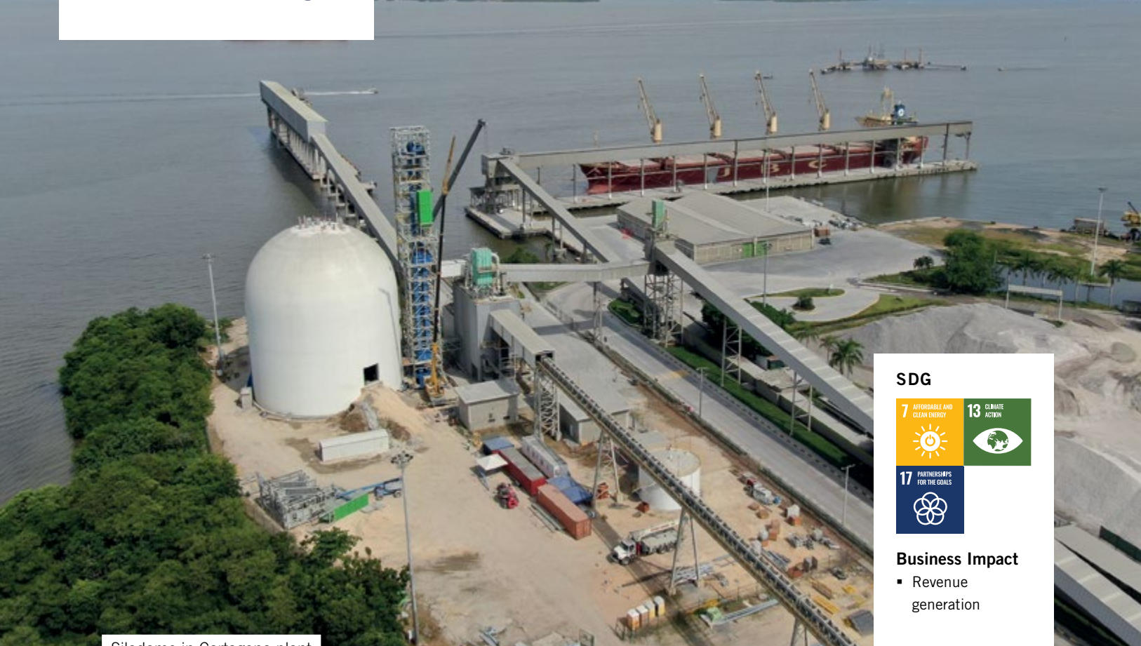
Silodome in Cartagena plant
