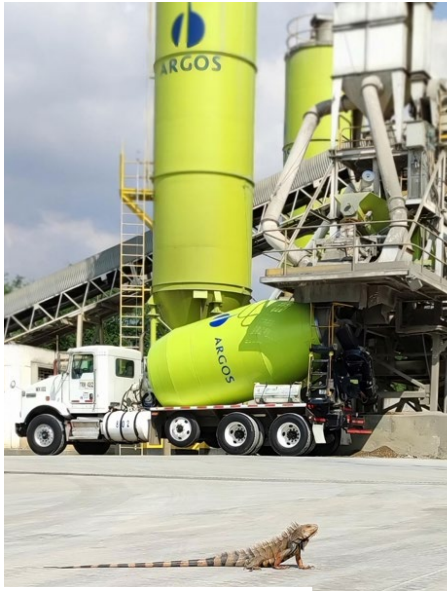
Concrete Plant (photo taken by employee Juan Carlos Villota)
