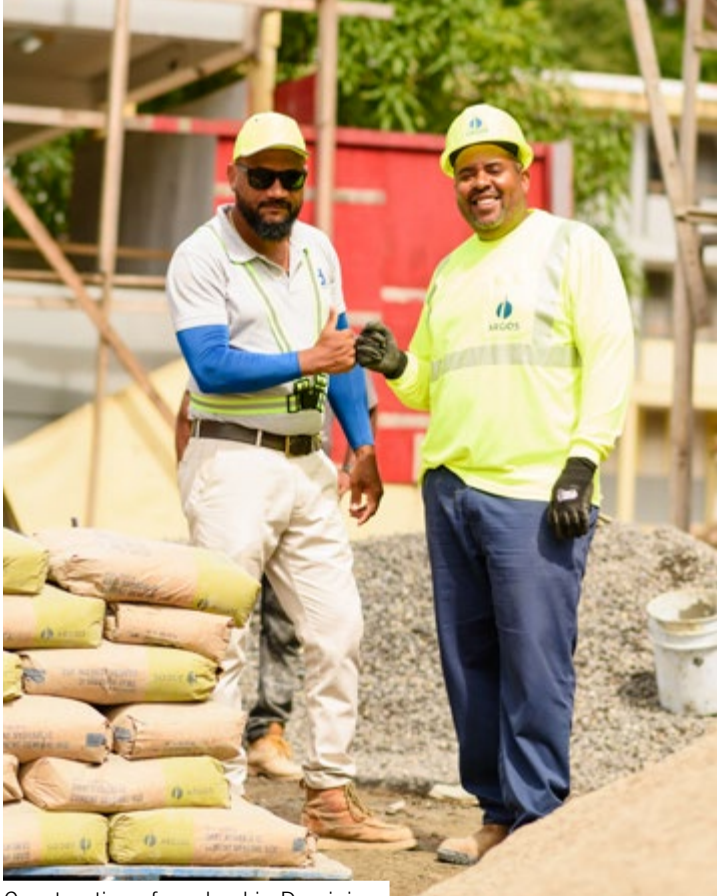
Construction of a school in Dominica
