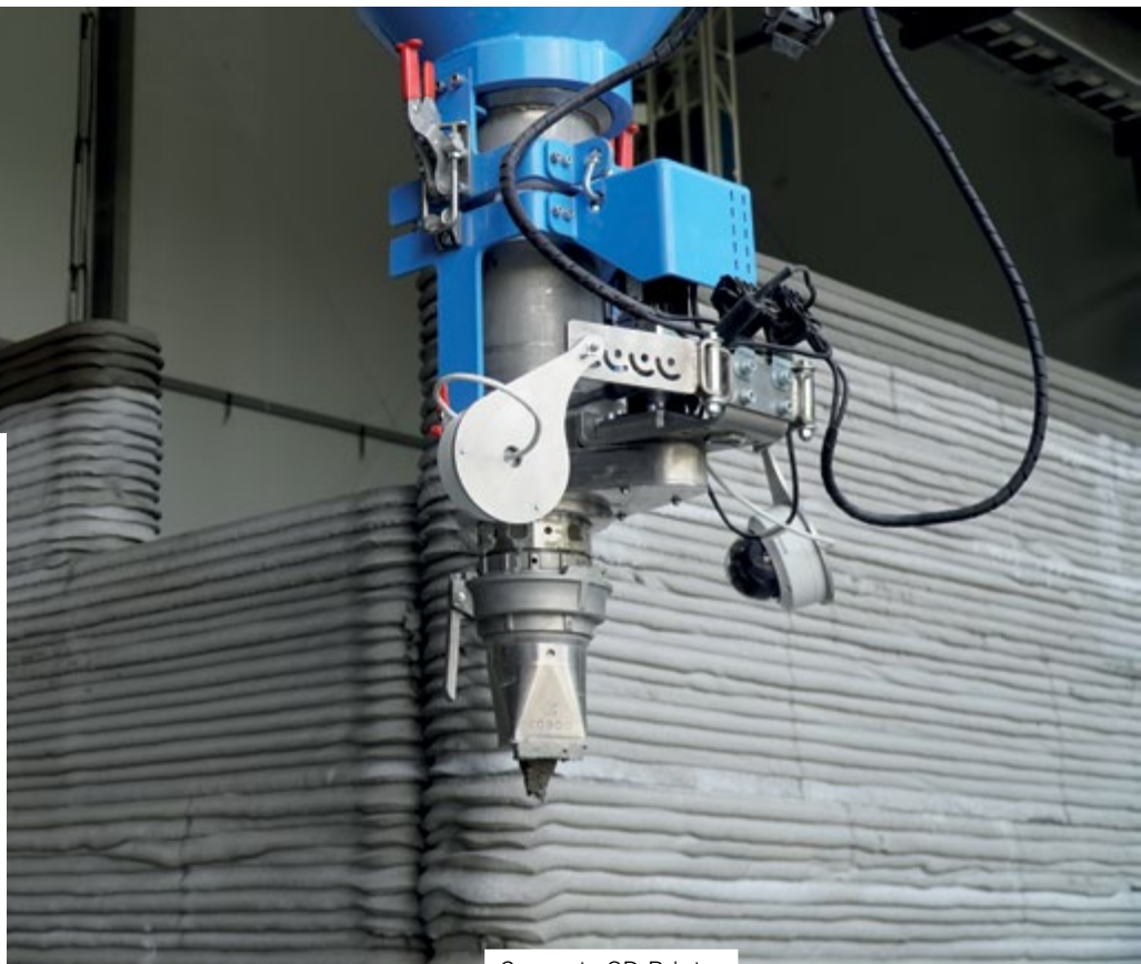
Concrete 3D Printer
