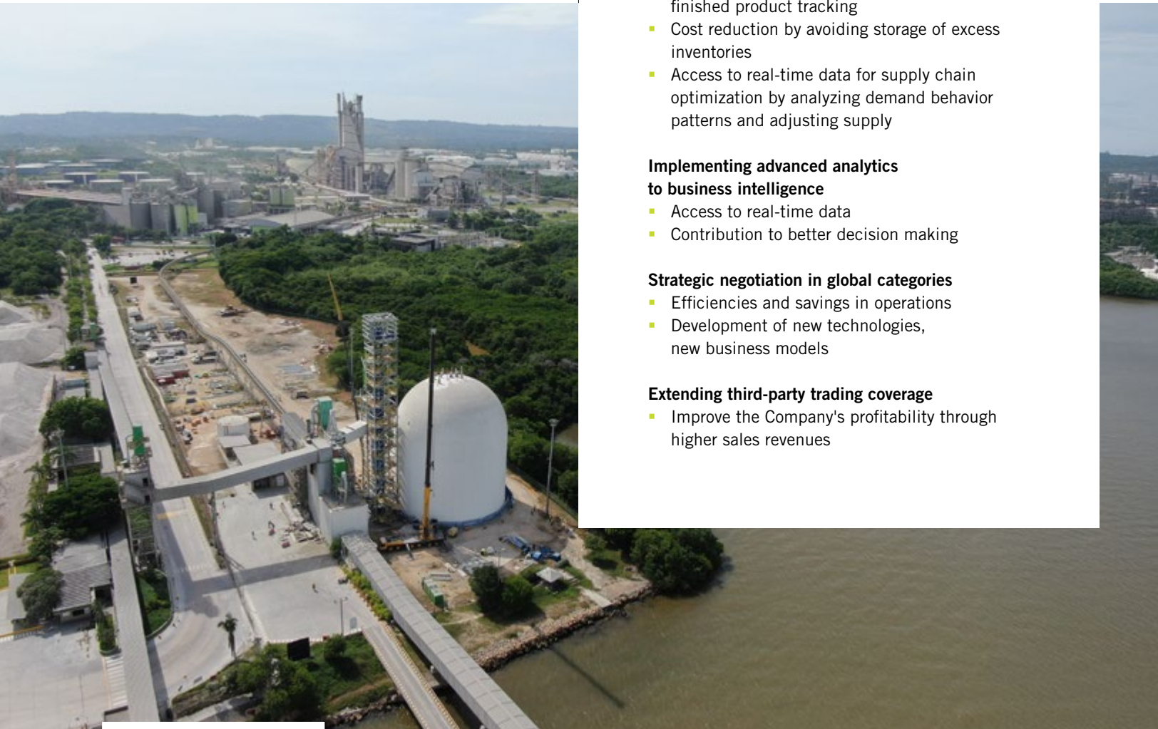
Silodome in Cartagena plant
