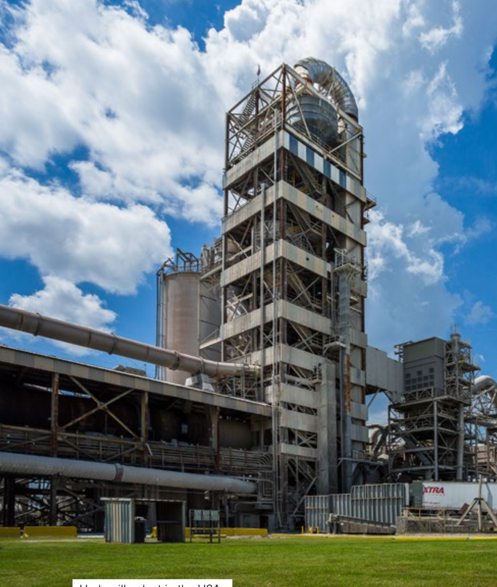
Harleyville plant in the USA.
