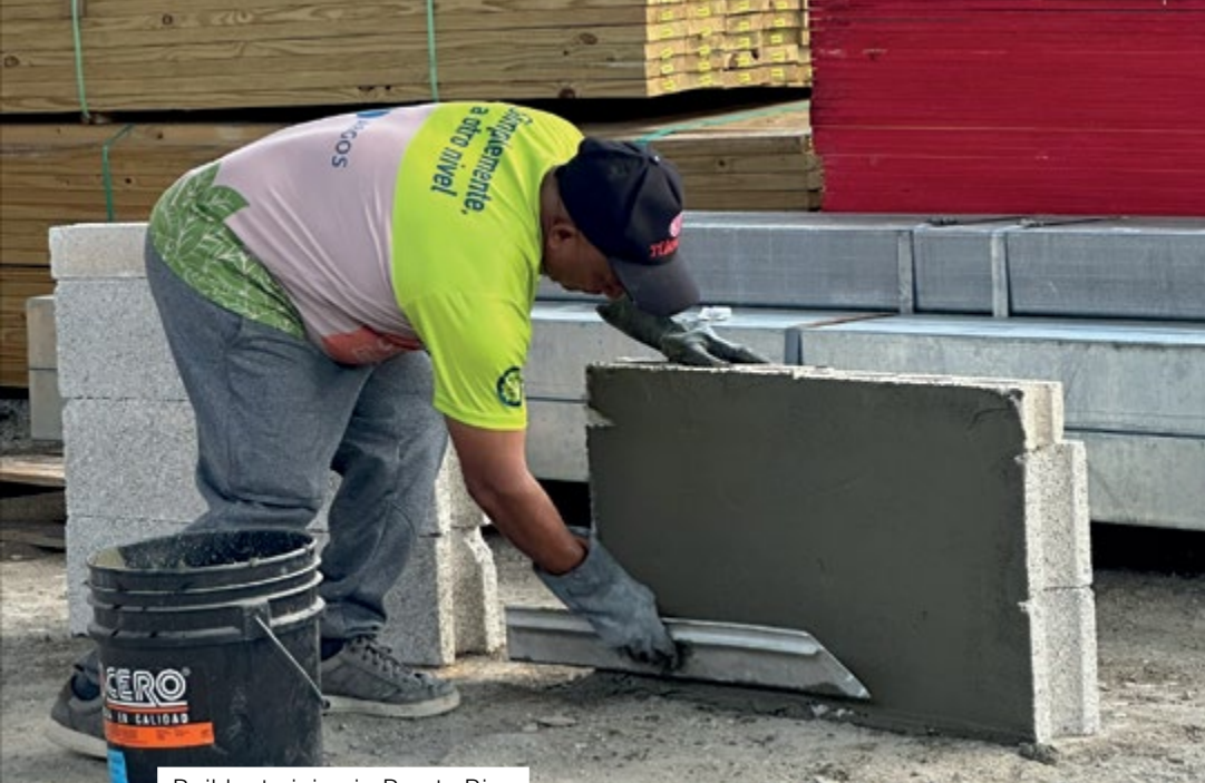
Builder training in Puerto Rico
