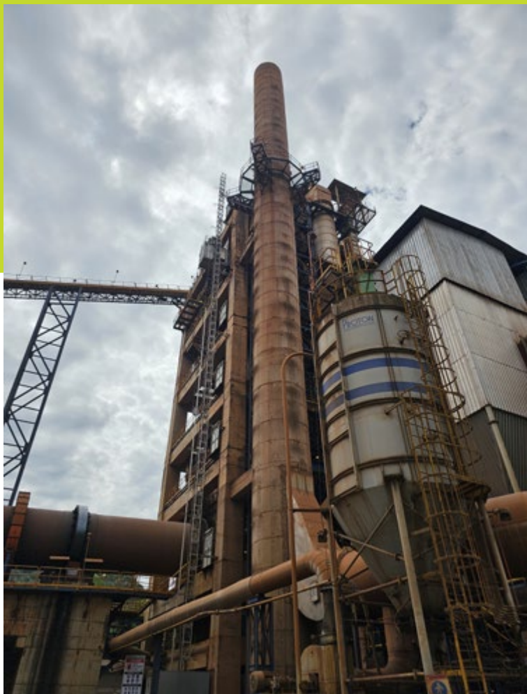
↑ Rioclaro Plant in Colombia
