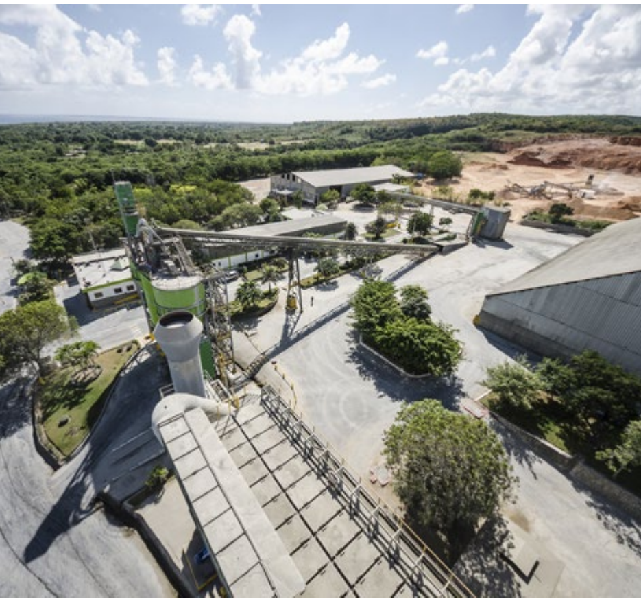
↑ Najayo Plant in the Dominican Republic
