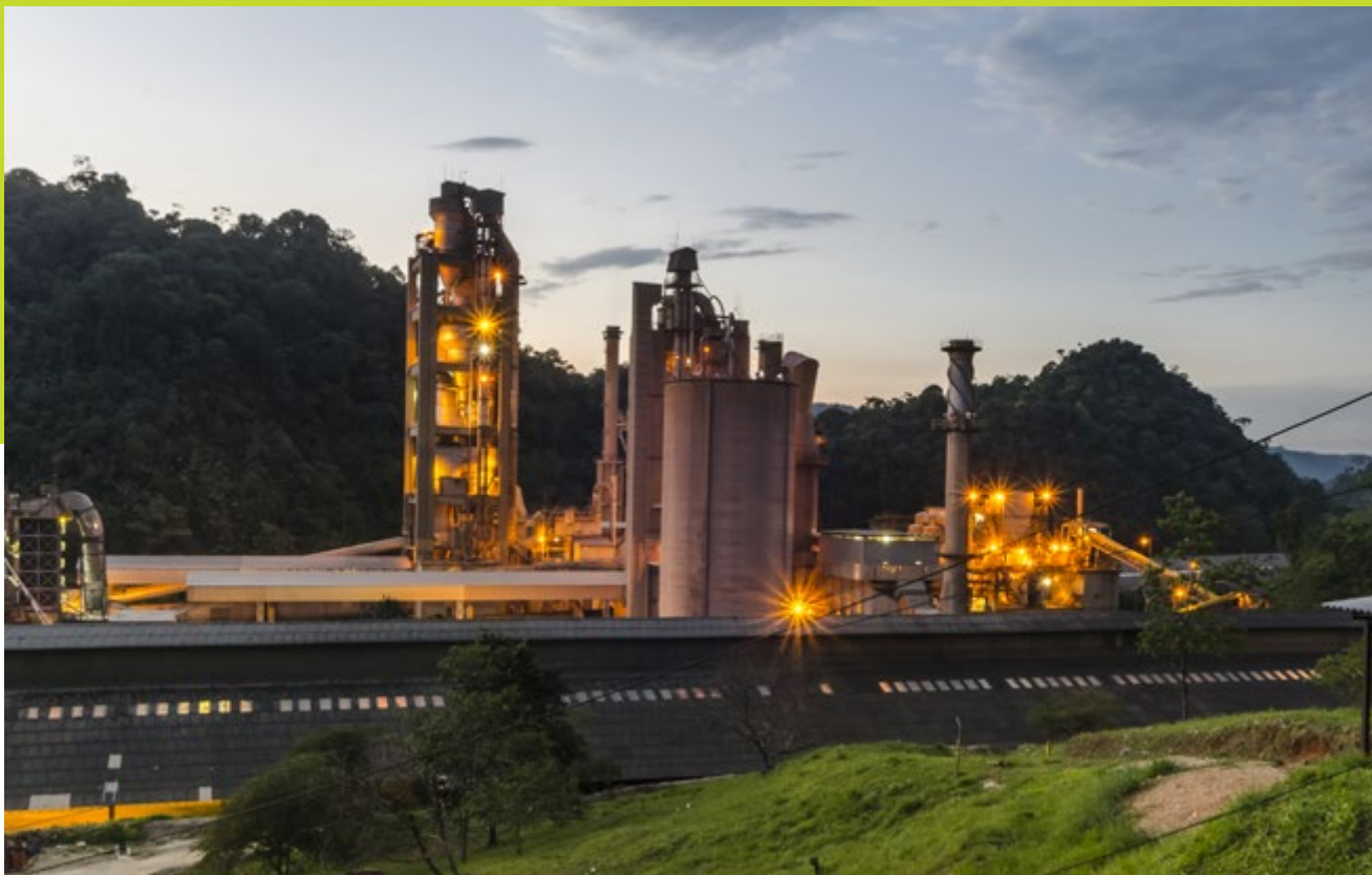
↑ Rioclaro Plant in Colombia
