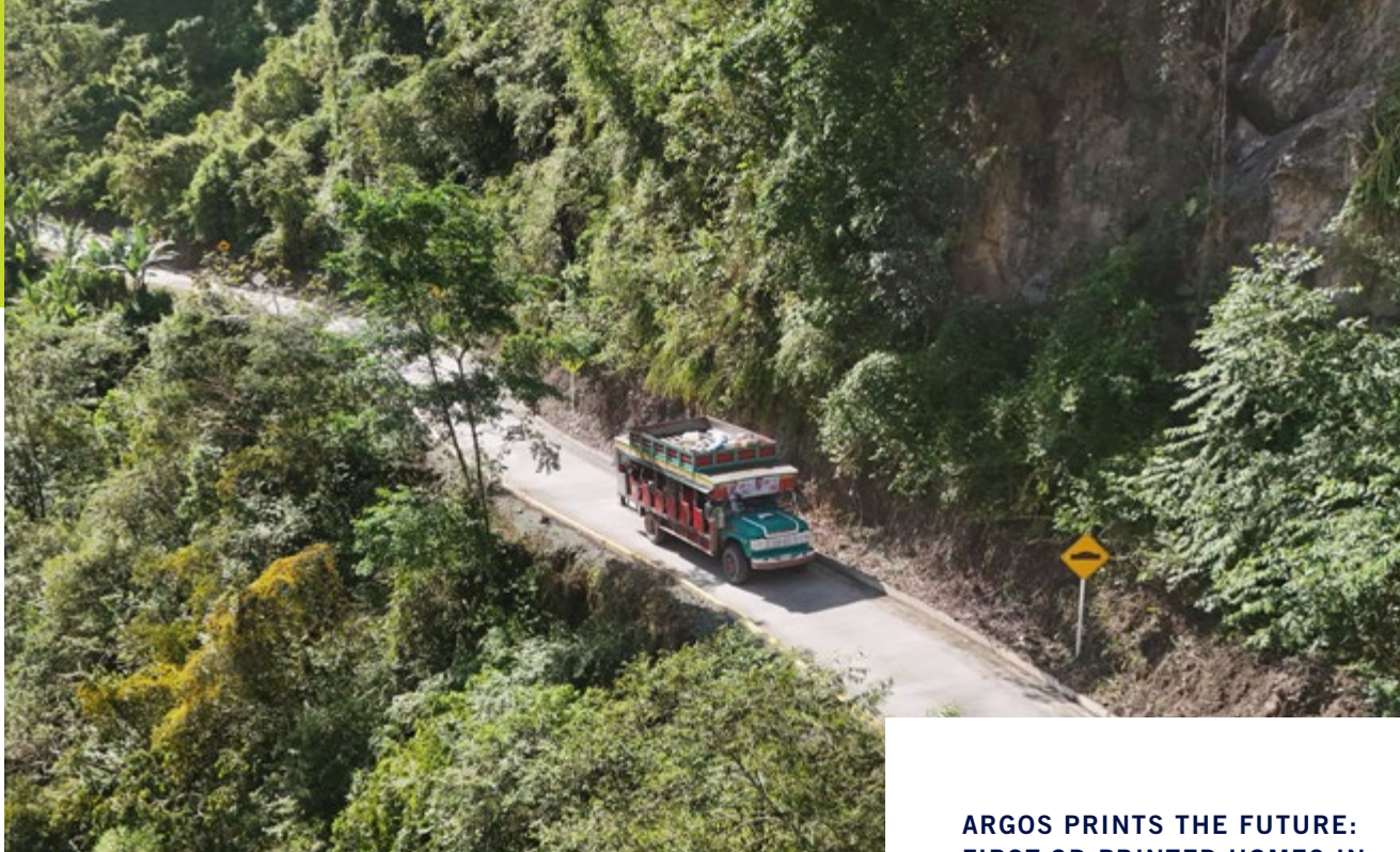
↑ Road in Dabeiba built through the "Work for Taxes" in Colombia
